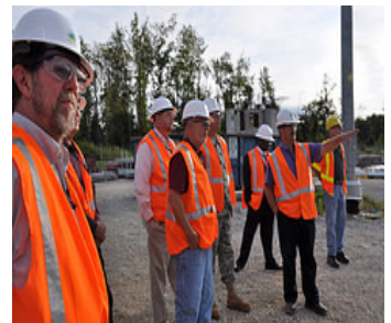
Members of the CDCAB touring the BGCAPP construction site in 2010.
