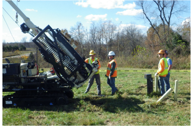
Crews working at the site of Monitoring Well No. 13.
